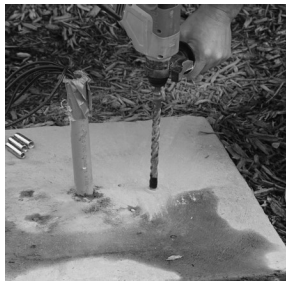
Figure 4.1 Drill Mounting Holes into Base
