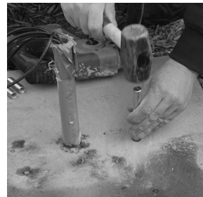
Figure 4.2 Tap in Drop-In Anchors
