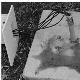
Figure 4.3 Feed Power Through Stub-Up
